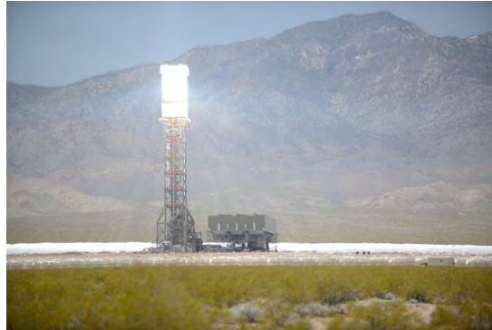
Ivanpah CSP Facility By Aioannides - Taken from side of the Road near I15 Previously published: None, CC BY-SA 3.0, https://commons.wikimedia.org/w/index.php?curid=25841974
