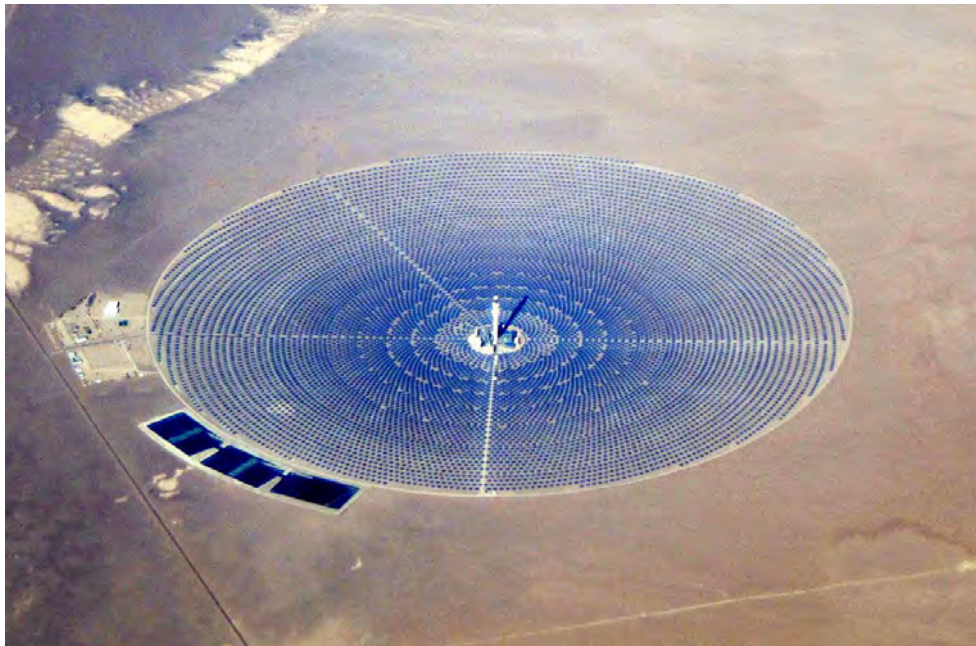
Crescent Dunes Concentrated Solar Power Facility. Source unknown
